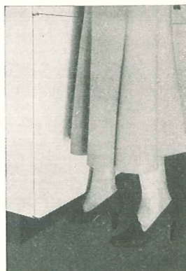
All base cabinets are constructed with a set-back, or recess, on the floor line to provide ample toe space.
